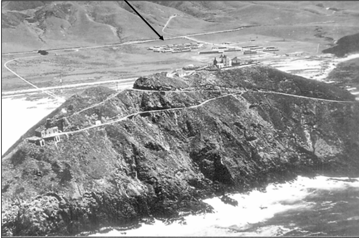
Historic Photo 4. Circa 1960 view of the Point Sur light station, with Moro Rock in the foreground and the NAVFAC seen behind. The Capehart housing neighborhood (arrow) is complete, without the Monterey Pine/Cypress windbreak at the top center of the image and shown by an arrow. (Courtesy: Point Sur State Historic Park General Plan , February 2004).
